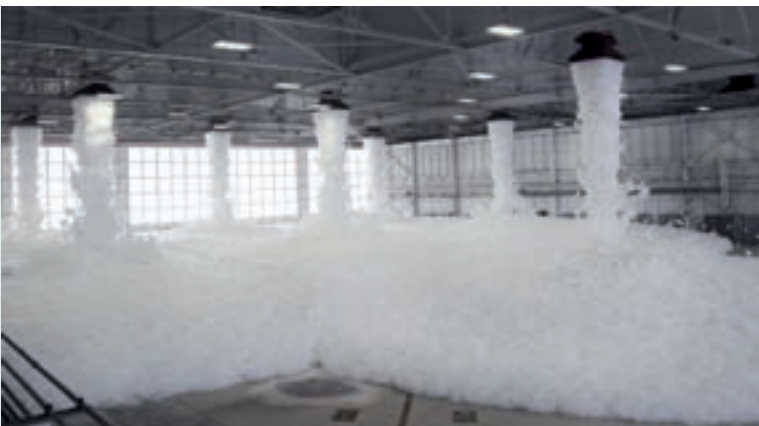
Figure 1: special protection extinguishing system – high-expansion foam in an airplane hangar.
